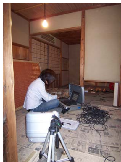
Fig.4 Structural Assessment: Micro-Tremor Test
