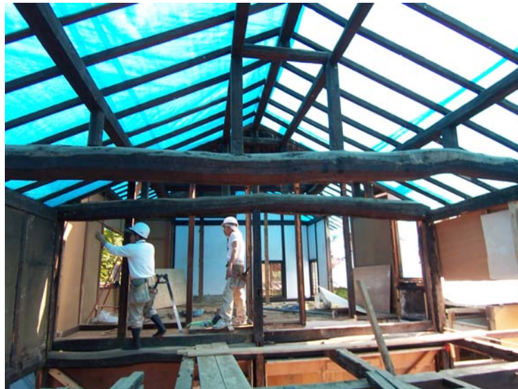
Fig.7 Student Construction Site for Timber Housing in Mino City
