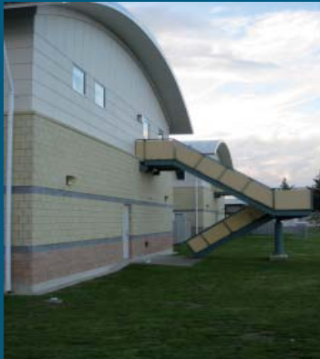
Waitakere Hospital, rear of ward accommodation ▲
